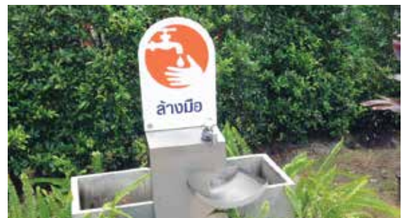
▲ Installing storages for rainwater and wastewater in order that they can be reused or recycled for watering plants and other usages, enabling water conservation.
